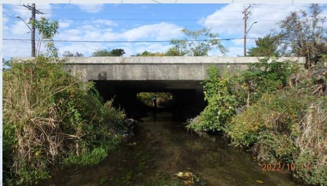
North elevation view of the culvert
